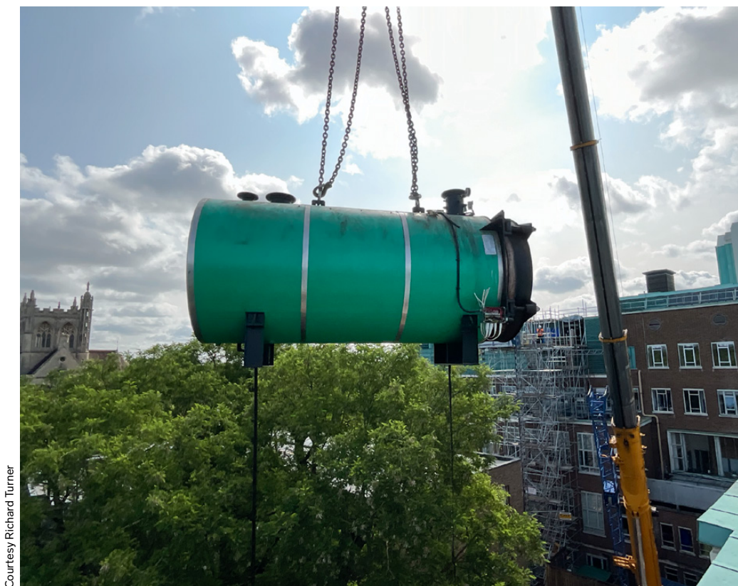
Above: Old boiler removal.
