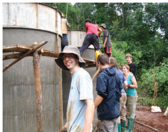
Right: A bucket chain for building the storage tanks
