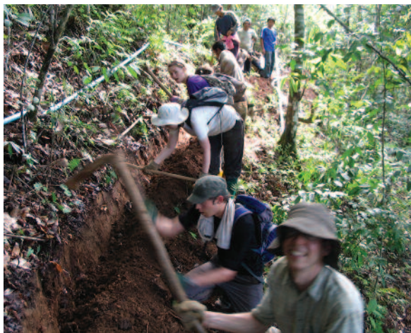
Digging in the pipes was hard work with a hoe!
